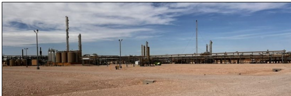
Pronto Midstream's Marlan Natural Gas Processing Plant
