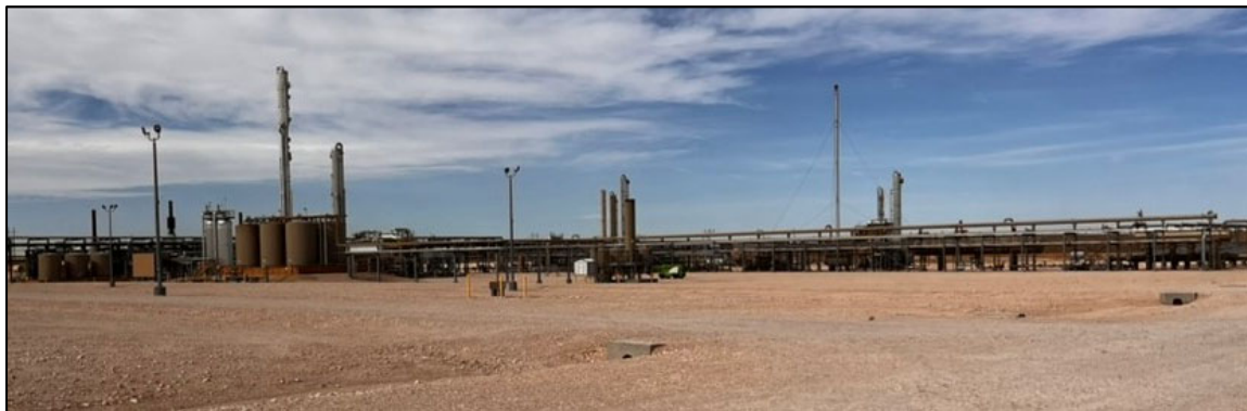
Pronto Midstream's Marlan Natural Gas Processing Plant
